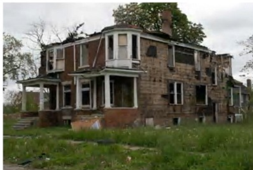
Abandoned house on Detroit's east side
